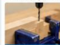
Clamp timber before drilling dowel holes.
