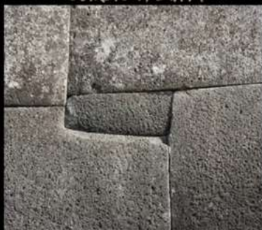
AHU VINAPU, EASTER ISLAND
