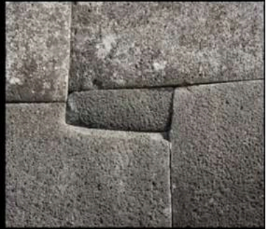
AHU VINAPU, EASTER ISLAND
